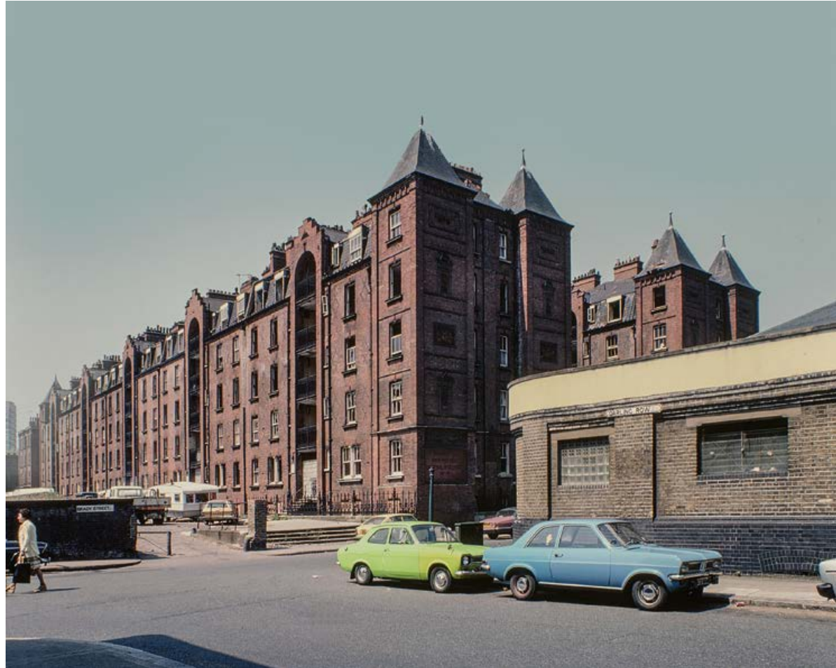
Brady Street Buildings, 1978
