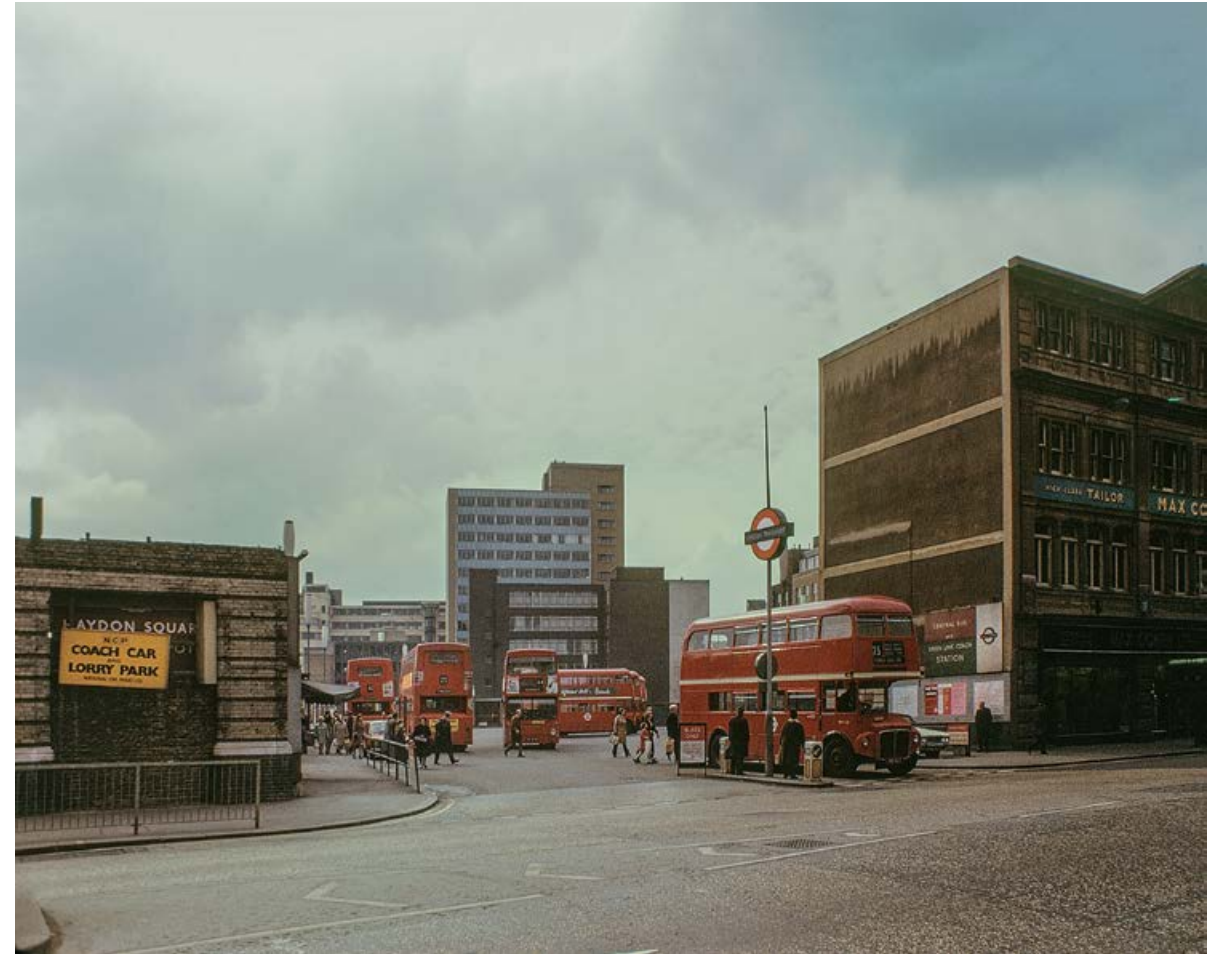
Aldgate High Street, 1975
