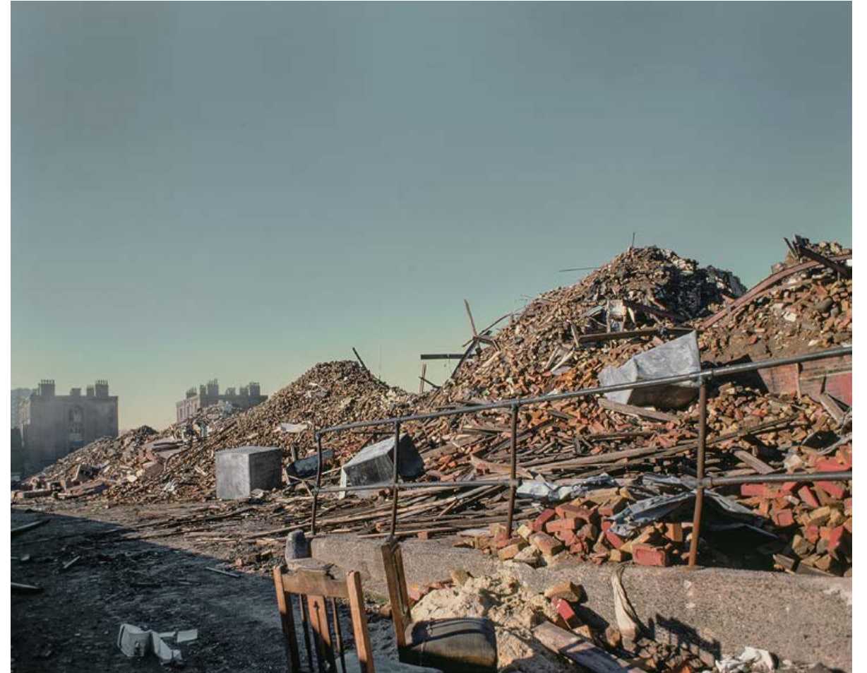
Brady Street Buildings, 1979
